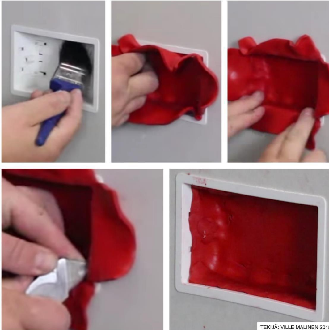
JOINTS FIRE PUTTY PAD PRO+ mouldable fire putty. Installation picture for socket boxes.
